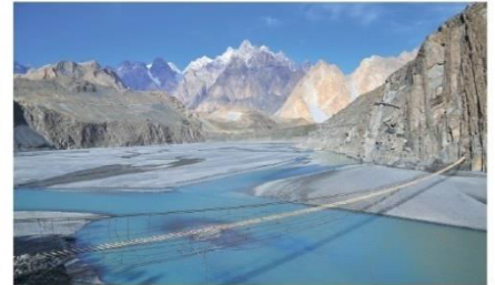
The Hussaini Hanging Bridge spans the Hunza River in Gilgit-Baltistan. MAINNOOR SAGHER
